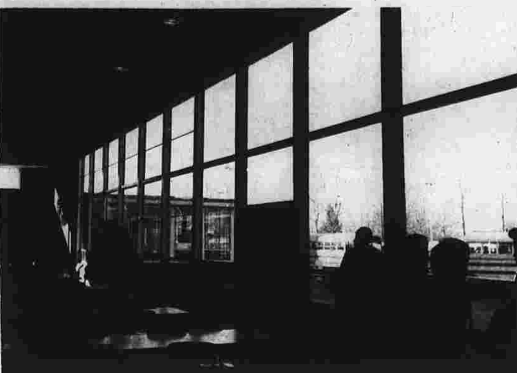
Two Miles of Windows The cafeteria at Manchester High School is the most blatant example of energy wasting design, with windows covering the length of one wall. The renovation plans call for extensive caulking and covering the windows with insulating draperies to keep in the heat. (Herald photo by Pinto)
